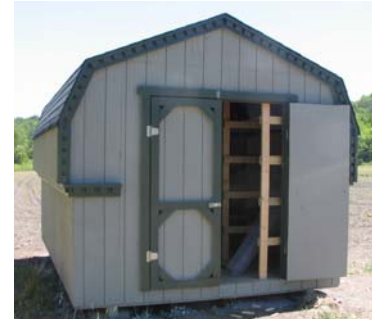
Figure 7: Converted 10' x 16' utility building..
