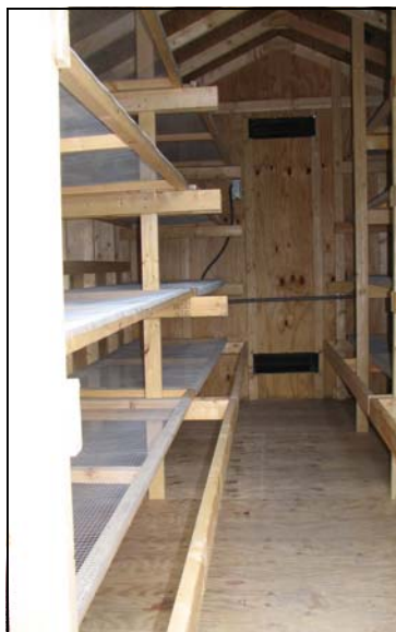
Figure 8: Unfinished frames with shelves installed.
