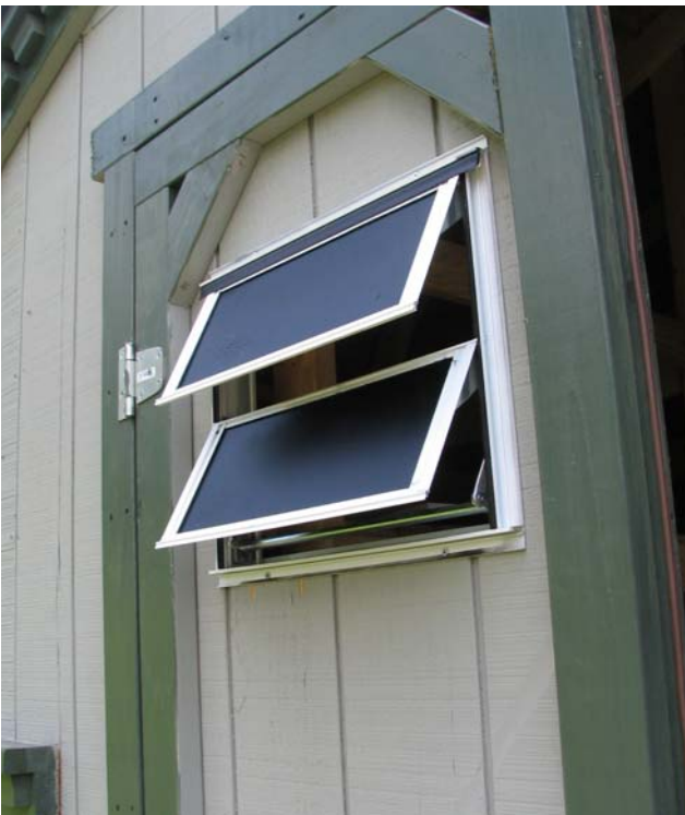
Figure 12: Window with screen and crank. Adjusting the opening of this window regulates the ventilation in the dryer.
