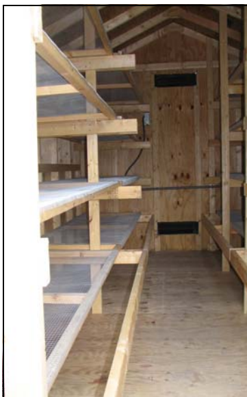
Figure 8: Unfinished frames with shelves installed.
